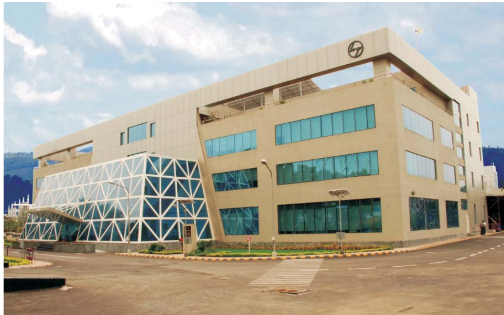
Switchgear Factory, Navi Mumbai
