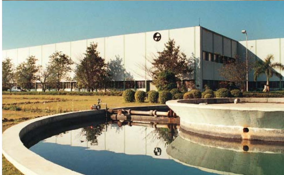
Switchgear Factory, Ahmednagar
